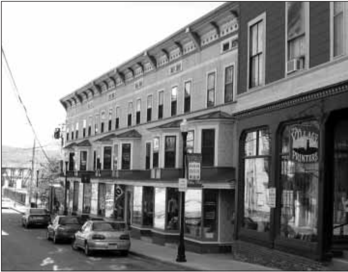
RACLT-owned Exner Block in Bellows Falls
