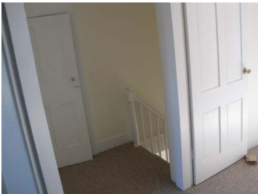
2 nd floor landing
