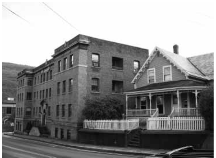
Abbott Block, 10 and 18 Canal Street
